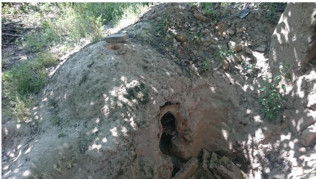
Fig. 7.1. Mr Ma's kiln: fire chamber; the chamber for loading pottery is on the right.
