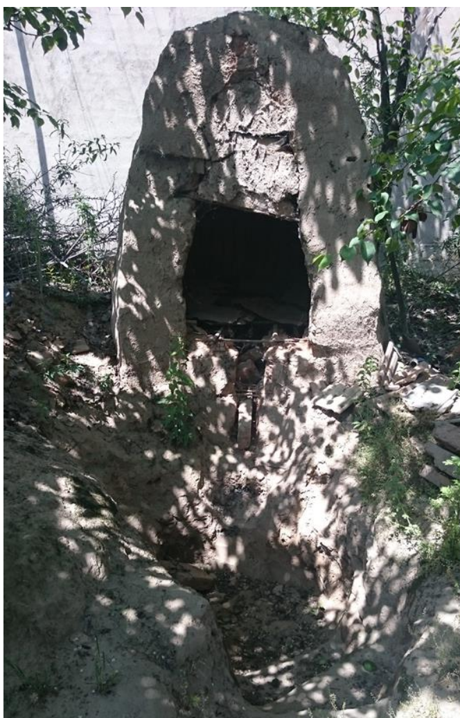
Fig. 7.2. Mr Ma's kiln: tall chamber for pottery loads; the firing chamber is on the left.
