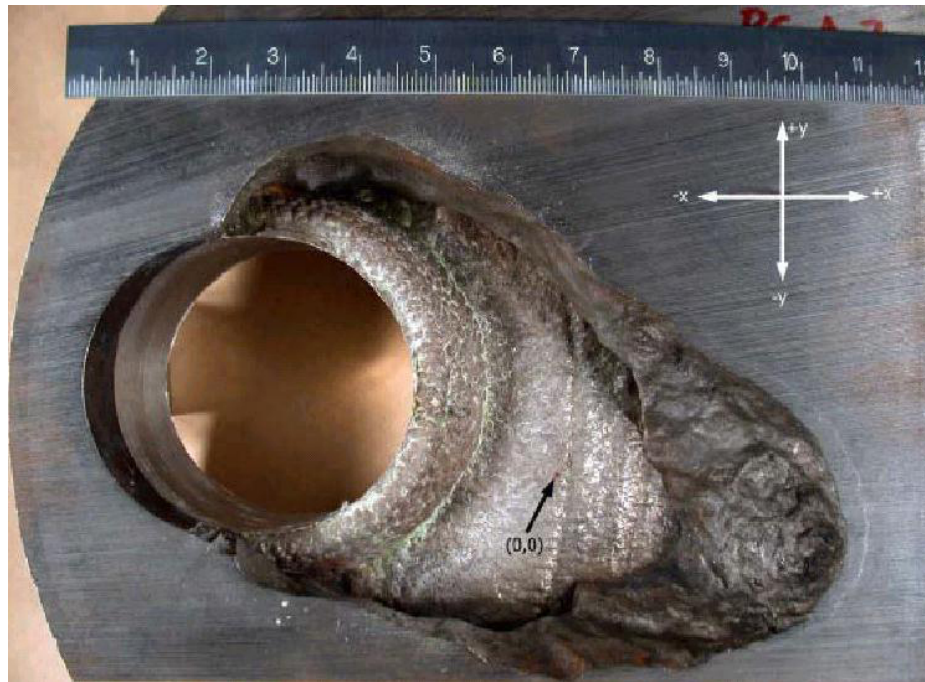
Figure 2: Top-view picture of the leakage and hole in the David-Besse PWR plant in Ohio. [11]
