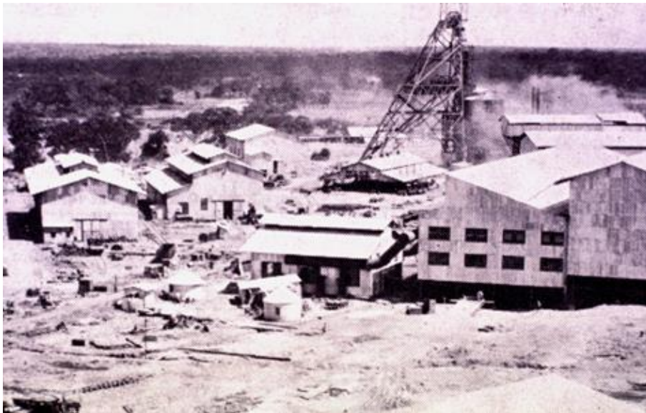
Figure 2.4: Surface plants and main shaft at Roan Antelope, circa 1930. A.W. Brooks, A History of the Discovery and Development of Roan Antelope Copper Mine .
