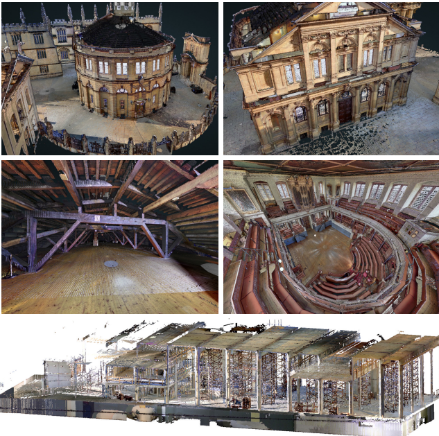
Fig. 7: Final point clouds built with the survey grade scanner. Top: Sheldonian theatre front and back exterior view. Mid: Sheldonian theatre attic and hall view. Bottom: Multi-level construction site side view.
