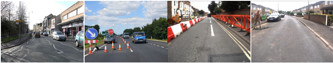
Figure 1.1: Typical complex road semantics (from left to right): worn out or ambiguous road markings, roadworks changing road layouts and worn tarmac with patched potholes.
