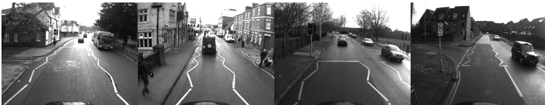
Figure 3.2: Zig-zag approach road markings lead up to a traffic light controlled pedestrian crossing.
