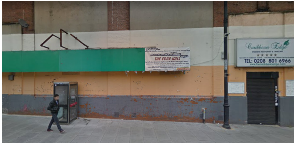
Figure 19: The Caribbean Edge, Bruce Grove, from street level.
