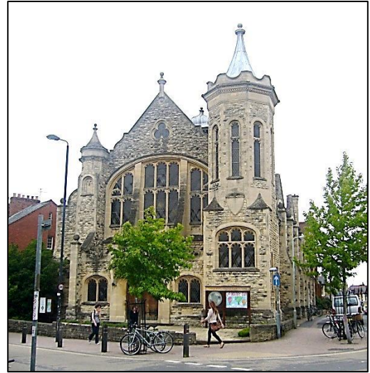
Figure 5.3: Wesley Hall, Cowley Road (2012) 14
