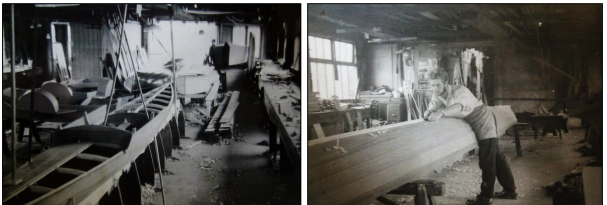
Figures 6.22 (left) and 6.23 (right): A first floor workshop at Grandpont Yard in the 1950s 156
