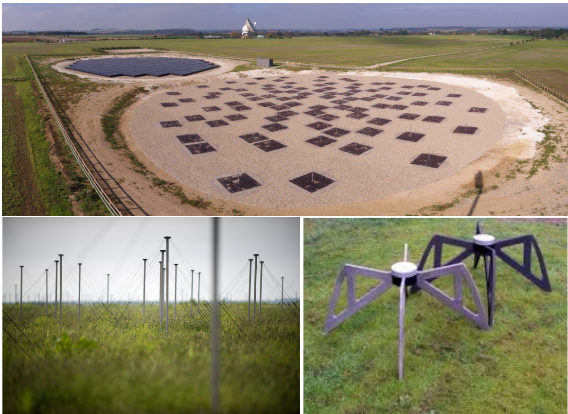
Fig. 2.1 Upper : The international LOFAR station at Chilbolton, UK formed with 96 single low band dipole antennas and 96 HBA tiles. Lower : Examples of the two types of antennas: LBA and HBA shown on the left and right respectively (picture credit: ASTRON).
