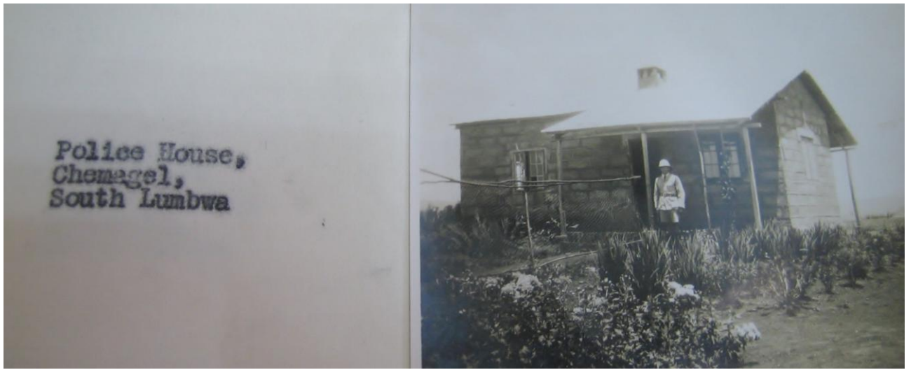
Station of the Colonial Police at Chemagel, South Lumbwa District, Nyanza Province.
