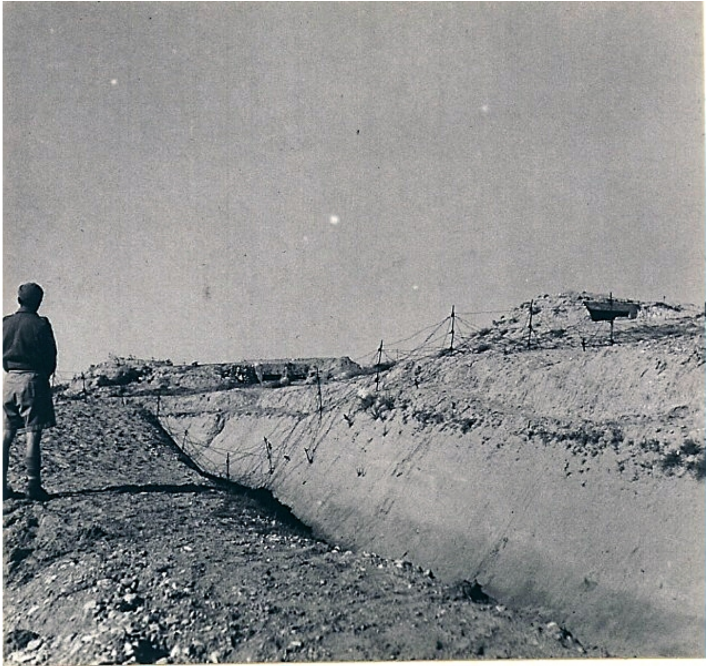
Figure 2: part of the Mareth Line after capture (IWM Photo Archive NA1469)
