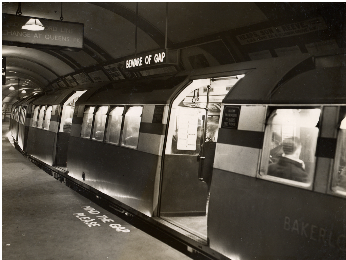
Fig.11 Topical Press, Waterloo Underground Station, Bakerloo Line, 17 January 1936, LTM, 1998/88454.
