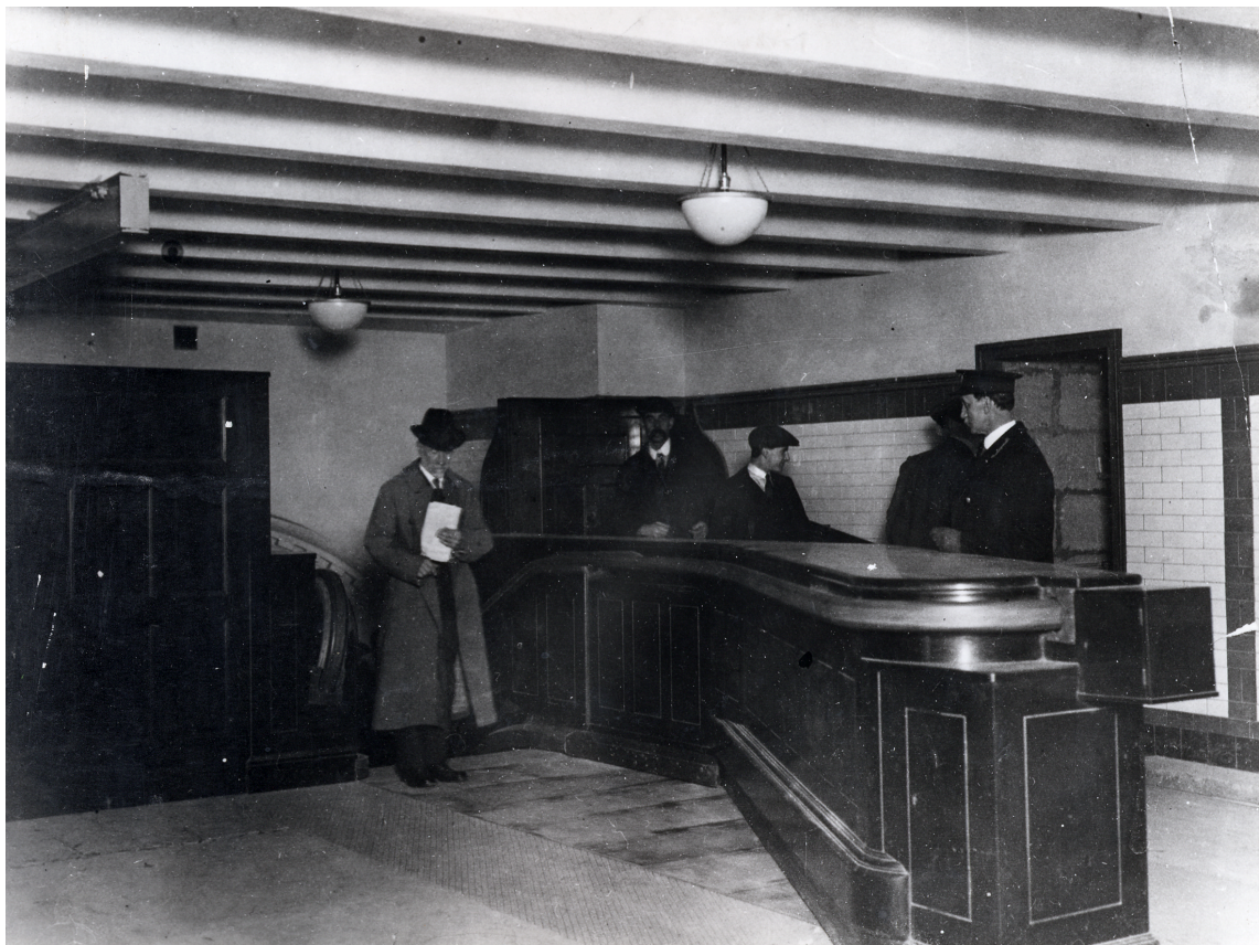
Fig.12 Upper landing of the escalator connecting the District and Bakerloo/Northern Line platforms at Charing Cross (now Embankment) station, c. March 1914, LTM, 1998/73649.
