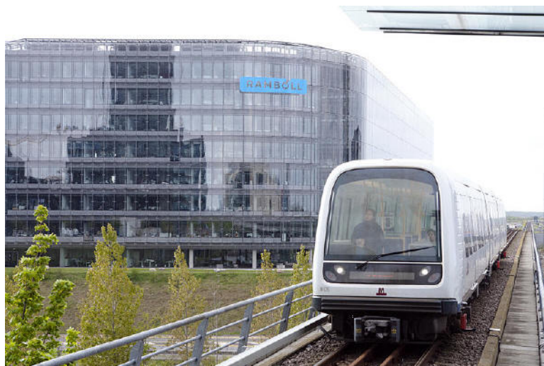
Figure 4: Copenhagen Metro on elevated tracks in front of Rambøll Engineering, Ørestad City. Source: Wikimedia Commons: Mdann52talk to me!
