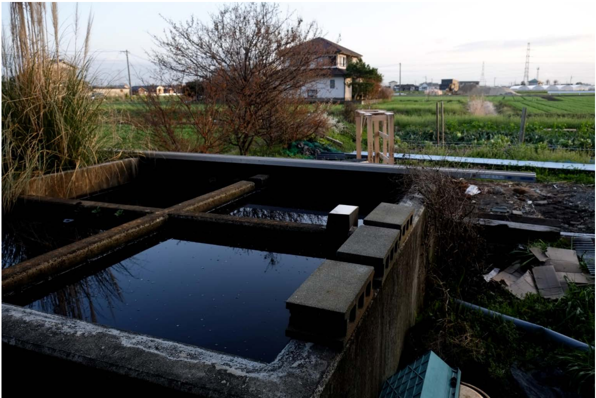
Top: Takarejima Senkou studio; Bottom: wastewater tanks with farmland beyond.
