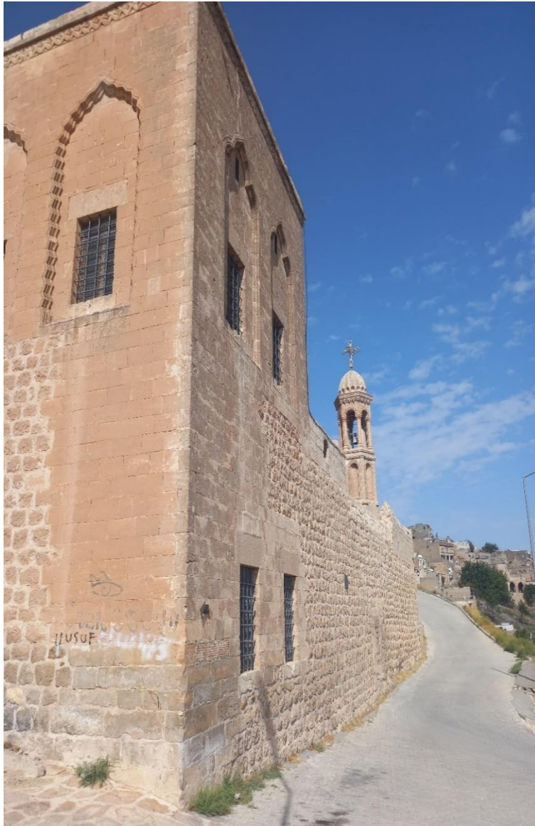
Figure 5: Church of St. Shmuni, Mardin, exterior (October 2023).
