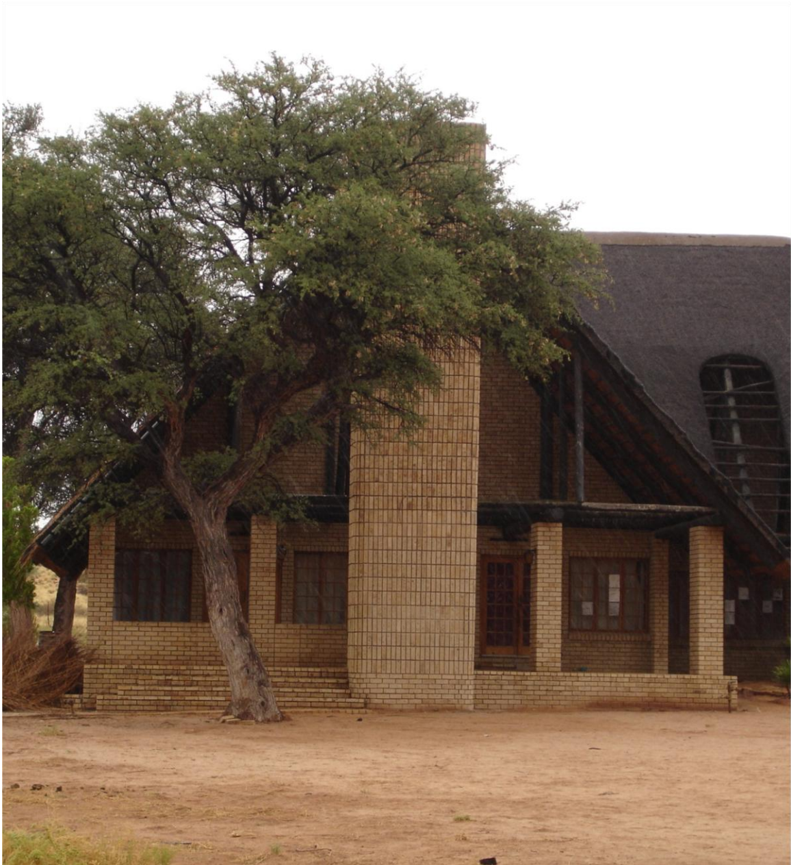
Figure 3.1: Formerly white-owned Scotty's Fort farmhouse, now in severe disrepair, that was 'grabbed' by the stock-farming Vaalbooi family during the disorganised rush on to the newly won #Khomani farms. Photo by the author.
