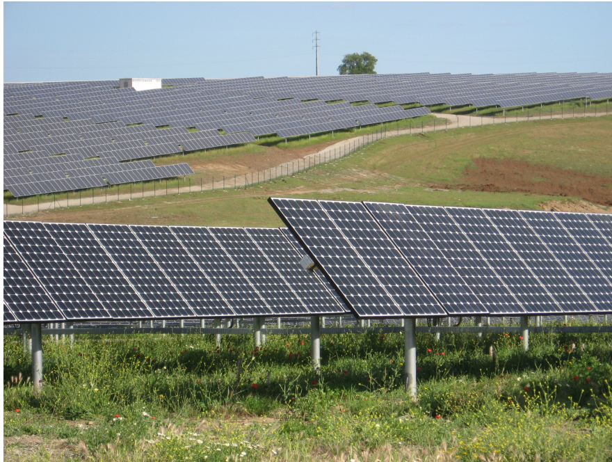
Figure 1.4: 11MW, 0.6km 2 (land area) solar power plant in Serpa, Portugal after [11].
