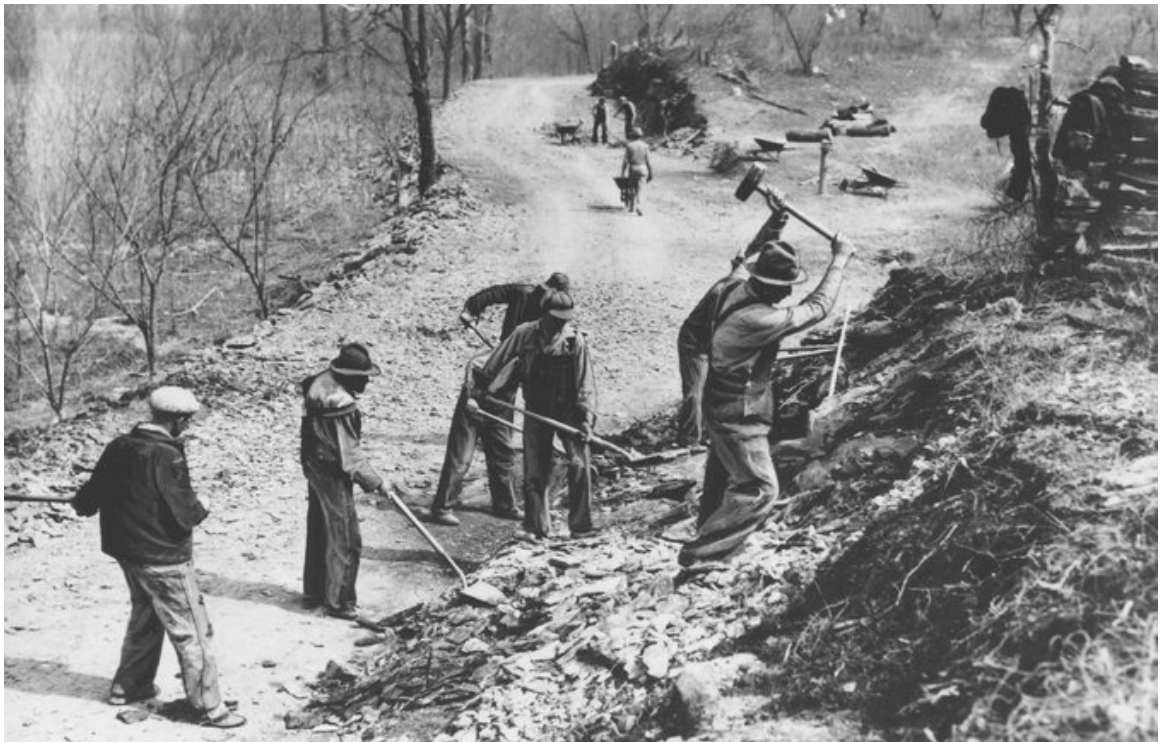
Figure 5.1: Work Progress Administration Workers Building a Farm-to-Market Road, Tennessee, 1936 (Unknown, 1936a)
