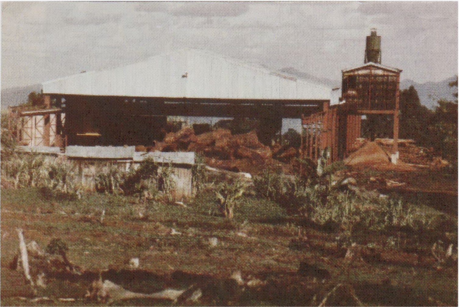
Appendix 2 Plate 4a: Nithi Timber Cooperative Society Sawmill Physical Plant and Log Storage.
