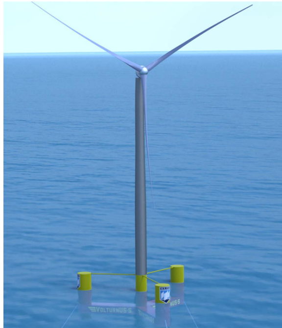
Figure 4.1: Rendering of the IEA 15 MW RWT and UMaine Voltturn-US platform from the Voltturn-US definition document [62].
