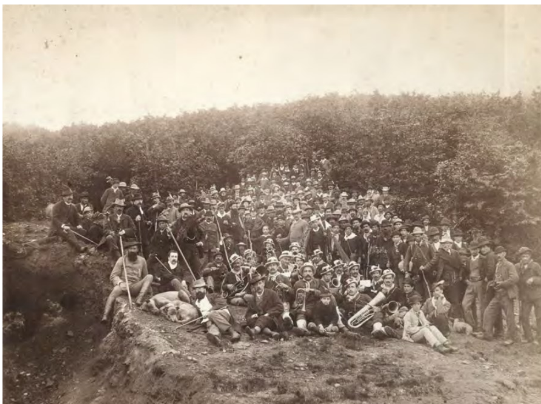
1. Celebrations at the Lake of Idols for the end of the excavations of 1838.
