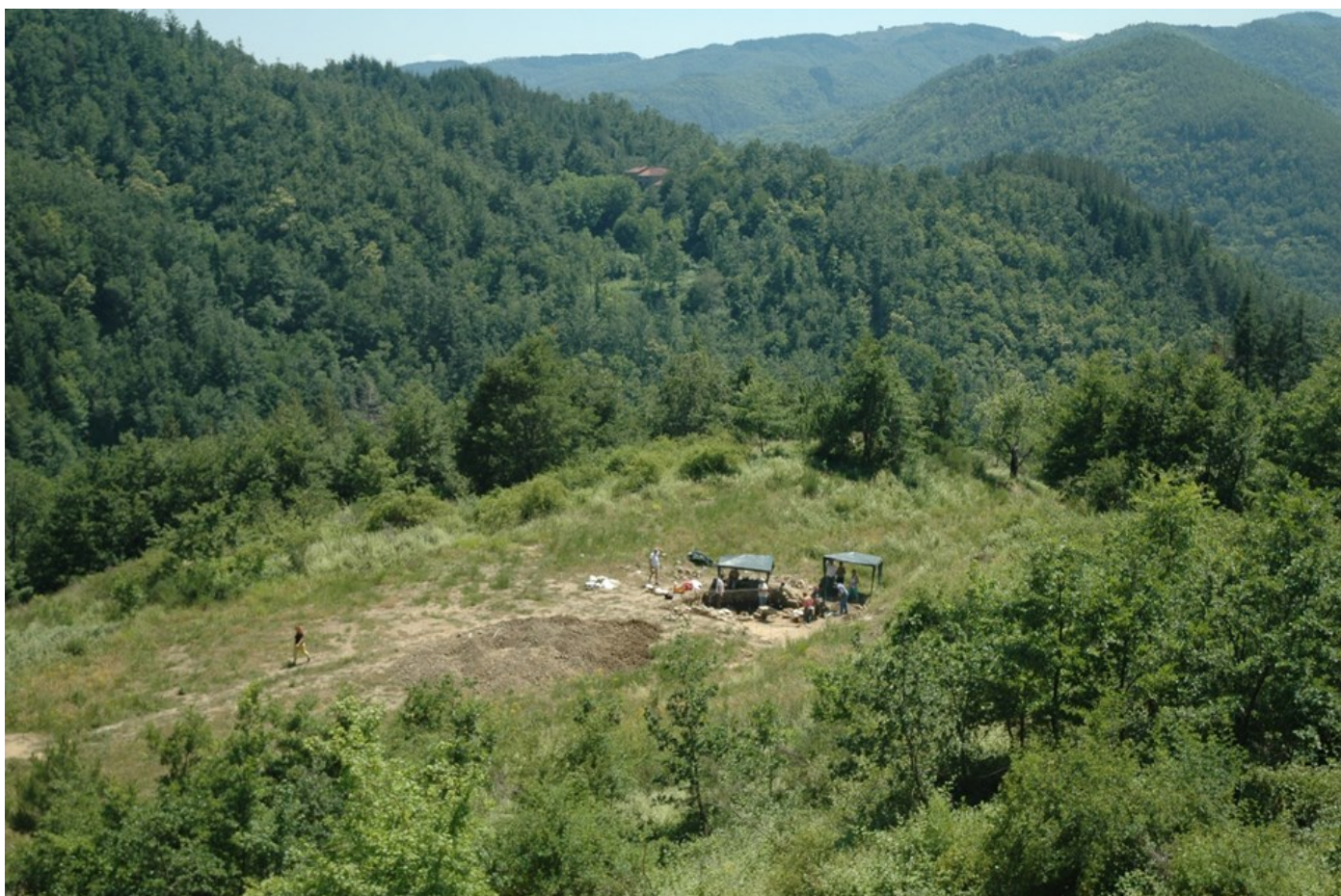
2. Excavation area at Serelli.
