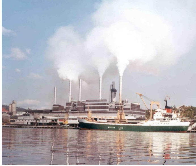
Figure 1.1: Elkem ASA’s silicon plant in Kristiansand (Norway, ca. 1970) releasing silica fume and other harmful gases into the atmosphere. Image provided by Elkem ASA [22].
