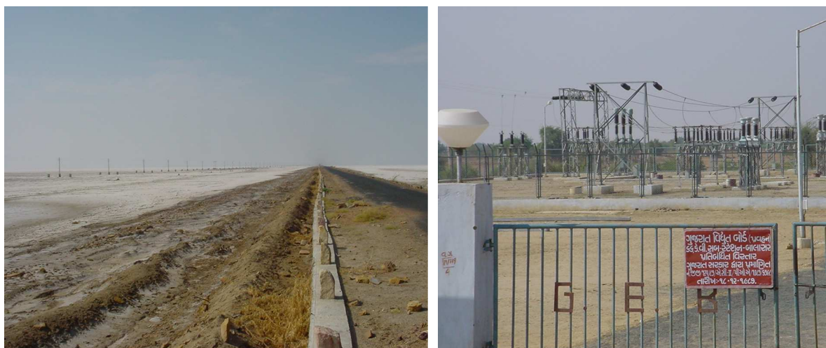
Figure 5-5: Transmission Line Across the Rann and GEB Substation in Balasar
