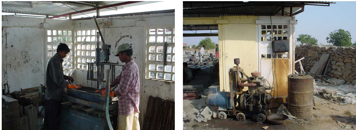
Figure 5-9: Concrete Parts Factory and 15 kW Diesel Genset, Khadir Island, Gujarat
