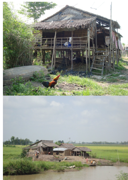
Top: Stilt house in Vinh Tri during dry season Bottom: House on dirt foundation in Vinh Tri during dry season
