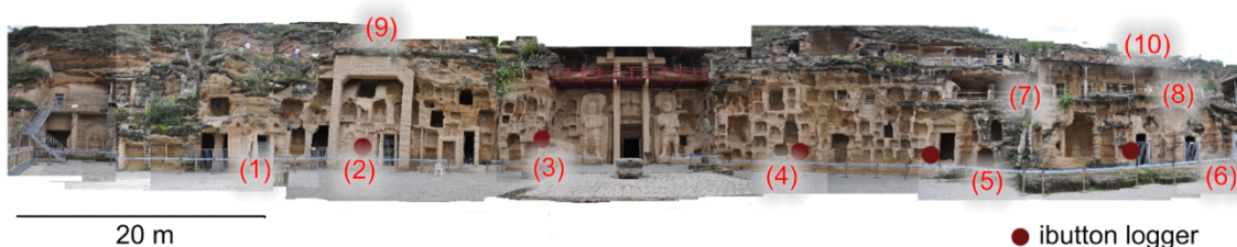
Figure 5.2. Salt extraction locations and ibutton loggers on NGT façade. [(1) niche 257, (2) niche 247, (3) niche 200, (4) niche 292, (5) niche 027, (6) niche 271, (7) niche 029, (8) niche 032, (9) north 3, (10) niche 035.]
