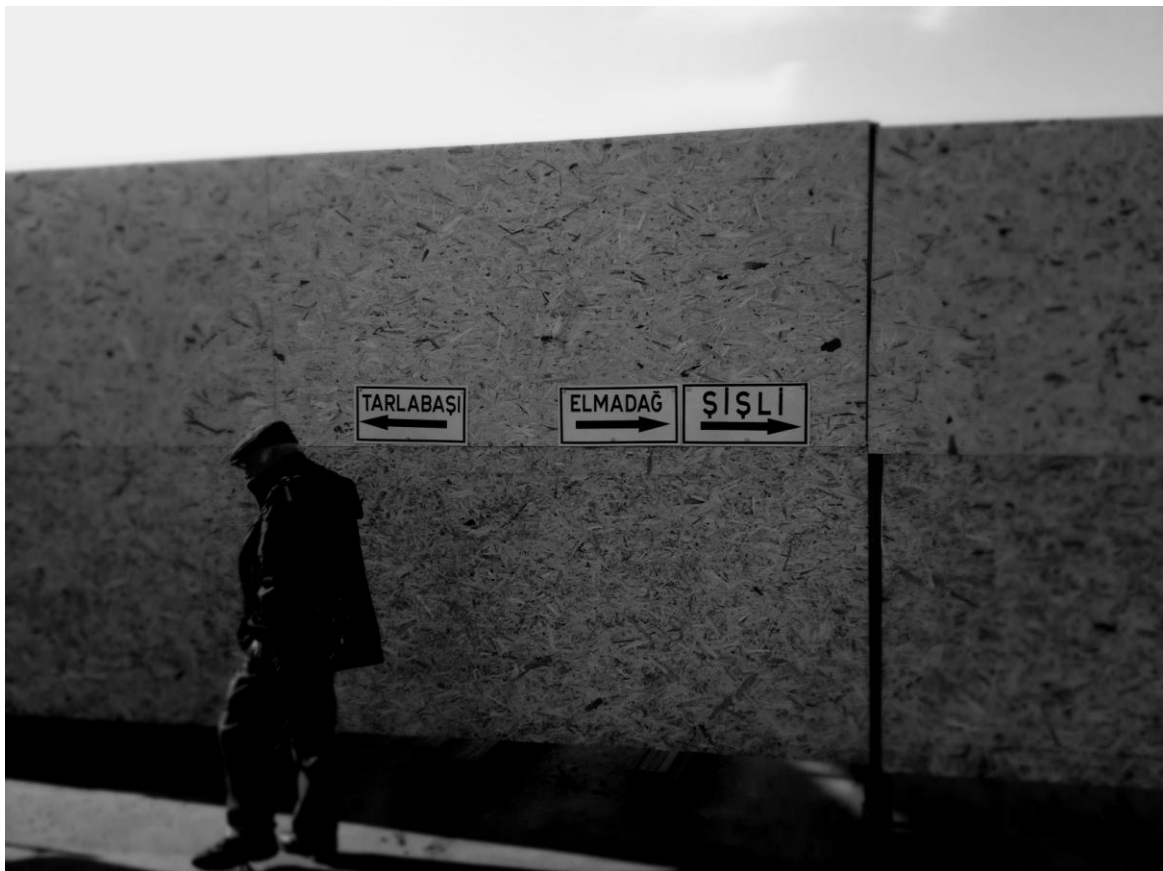
Figure 8.11 Pedestrians are forced to walk along the construction site with very little direction given to them Photo: Eda Beyazıt
