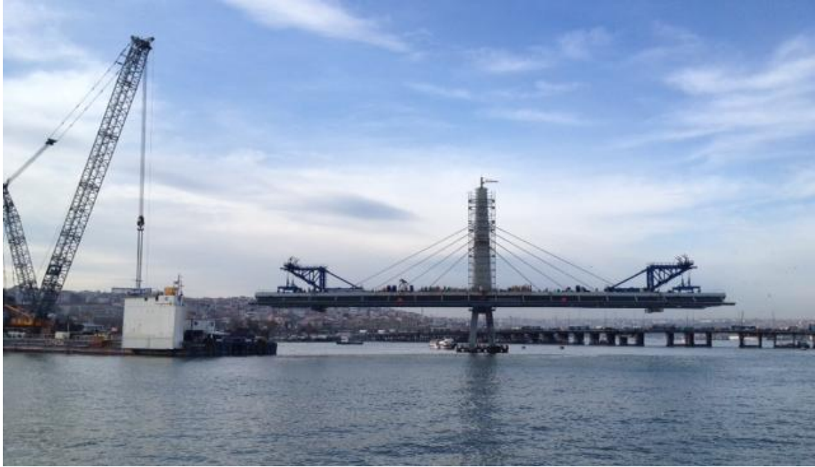
Figure 8.9 Picture showing the construction of the GHMB Photo: Eda Beyazit
