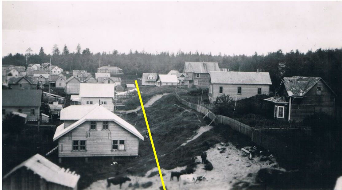
Figure 3.1. Picture taken by A2 (Old Massett), dated 1945-1950, showing where the current road (Raven Road) is, which currently goes right along the edge of the beach and the houses. Thus, all the houses and land to the left of the line have been lost, and it is now only beach.
