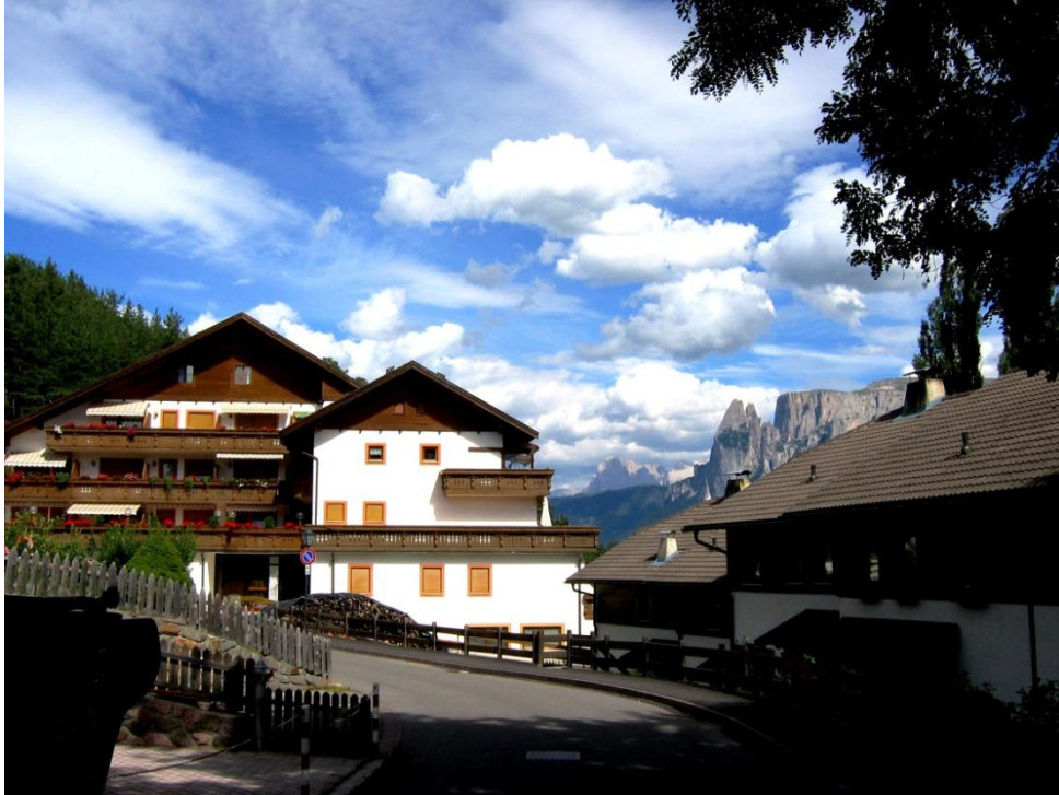
Figure 1.2 This is typical of South Tyrolean architecture, which is similar to Austrian house dwellings.
