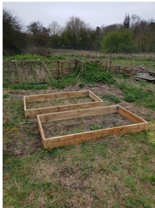
Figure 14: Constructing raised beds
