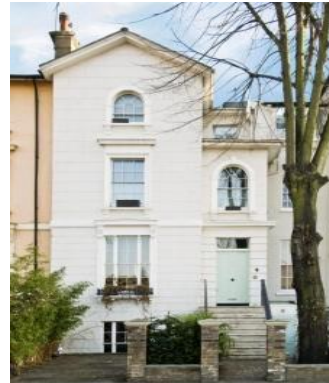
7.29 Westbourne Park Villas, Bayswater, west London
