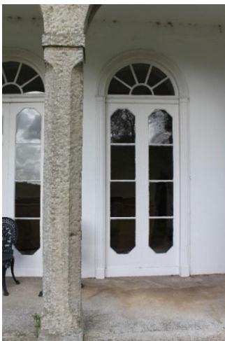
4.28b Loggia and detailing
