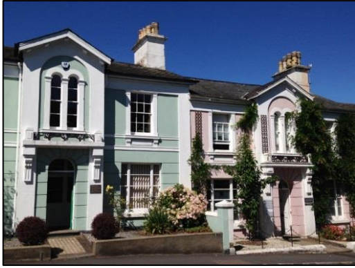
7.49 Devon Square, west side
