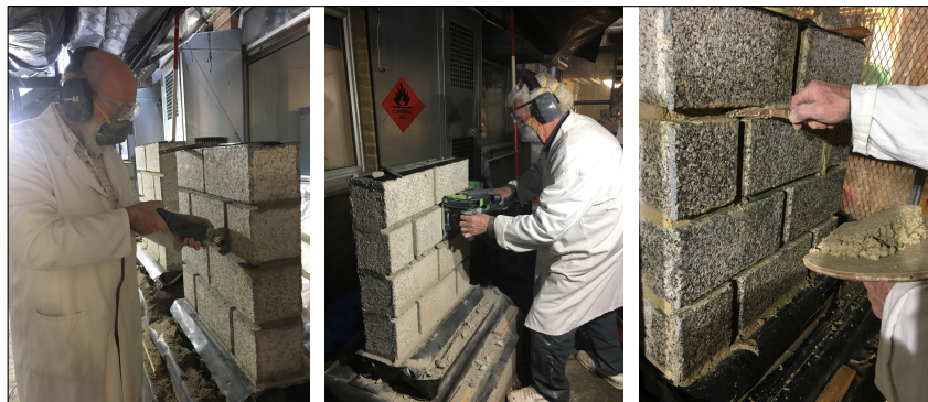
Figure 6.2. Removal of the former mortar joints and repointing.
