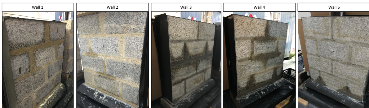
Figure 6.6. Visual assessment of the back of the test walls after 3 h of spraying and 6 h of evaporation (T=6 h). Water ingress visible through the bottom joint in all wall was not measured.
