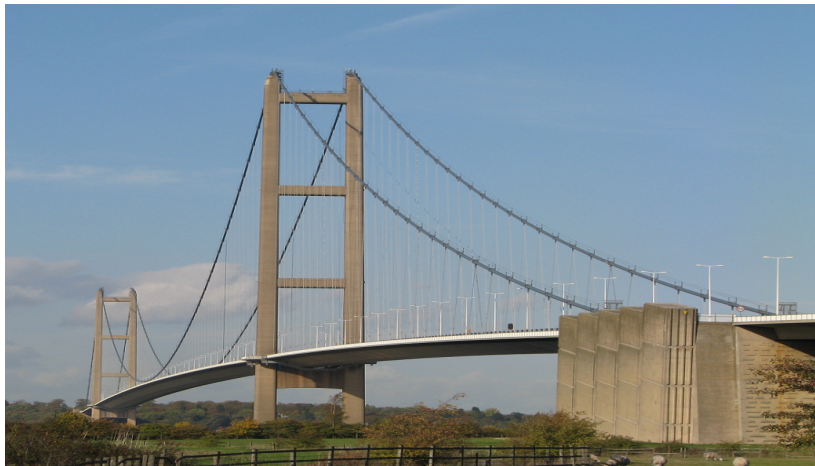
Figure 3.5 View of the Humber Bridge [157].
