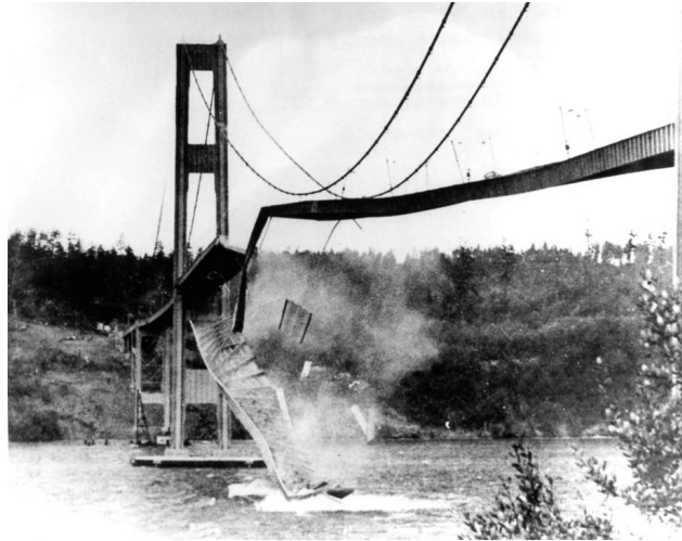
Figure 1.4 Collapse of Tacoma Narrows Bridge (courtesy of WSDOT).
