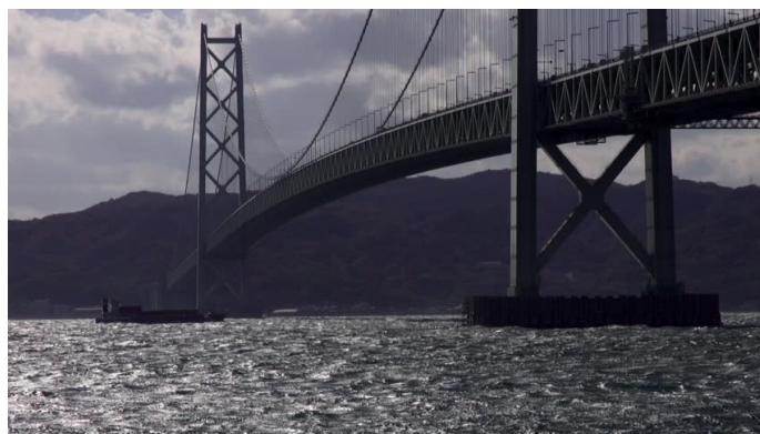
Figure 1.1 Akashi Kaikyo Bridge.
