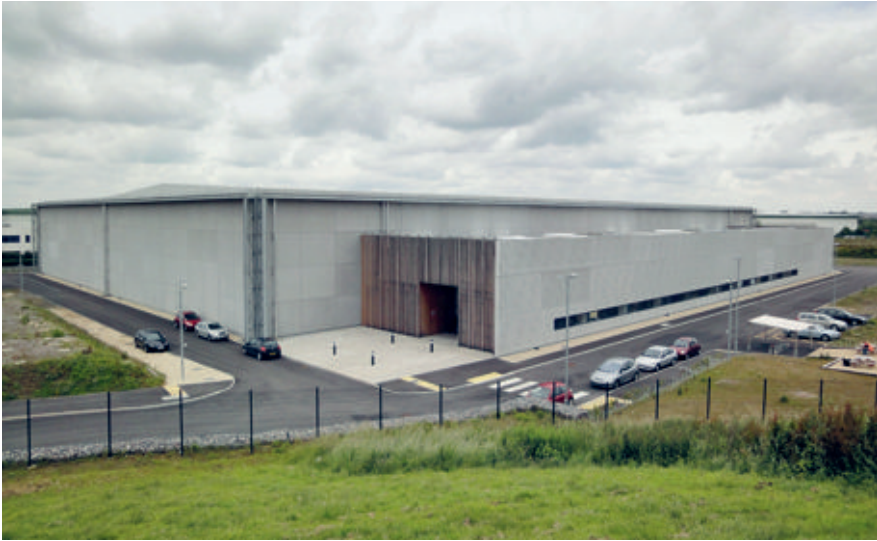
Figure 6.2: The Book Storage Facility from the south
