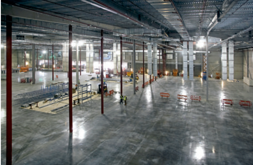
Figure 6.1: The Book Storage Facility under construction
