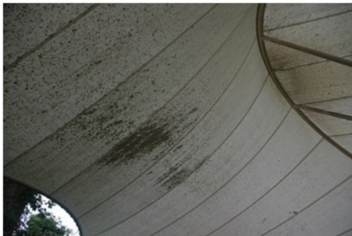
Figure 4.8: Dirt patches on the shelter membrane in October 2012. Image: C. Cabello-Briones
