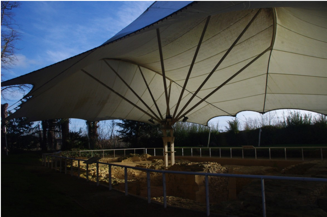
Figure 4.1: Open shelter built over the Bishop's Palace remains at Witney (Oxfordshire, England). Image: C. Cabello-Briones
