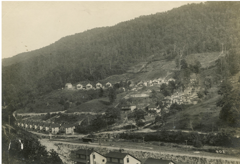
Figure 2.1: Image of homes built for coal miners in Jenkins, Kentucky “Jenkins from County Road, 1914 June 5”, Guide to the Jenkins, Kentucky Photographic Collection, 1911-1930, undated, University of Kentucky Special Collections Research Center.
