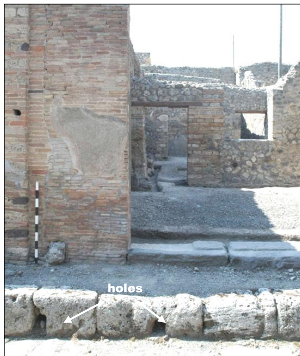
Figure 53B. The curb at the entrance to Unit IX.3.13 is pierced by two holes. The hole on the right is connected to the channel deriving from Room 70 (see fig. 14). Photo: T. Tuukkanen/ EPUH , 2010.
