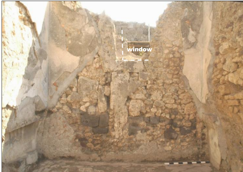
Figure 18A. The height of the window in the E wall of Room 52 (Unit IX.3.1-2) has been elevated thanks to the lowering of the floor level. Photo: M. Mustonen/ EPUH , 2006.
