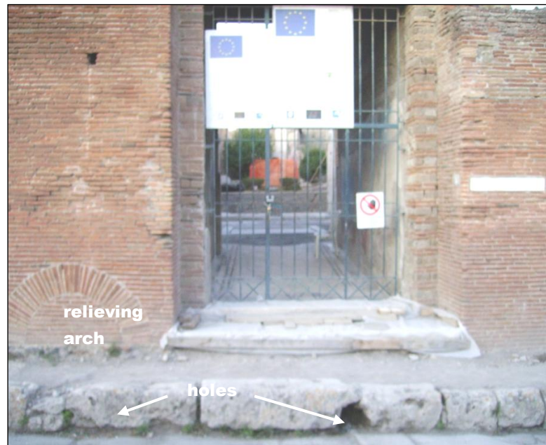
Figure 54A. The curb at the entrance to Unit IX.3.5/24 is pierced by two holes. Photo: author, 2008.
