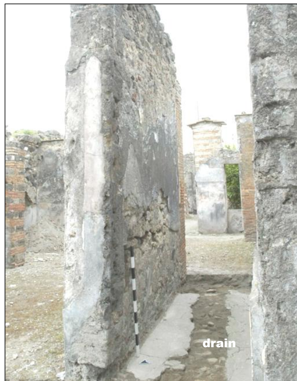
Figure 54B. The cover of a channel running N from Room 41 through Room 34 in Unit IX.3.5/24 had been exposed by AD 79. Photo: T. Tukkanen/ EPUH , 2005.
