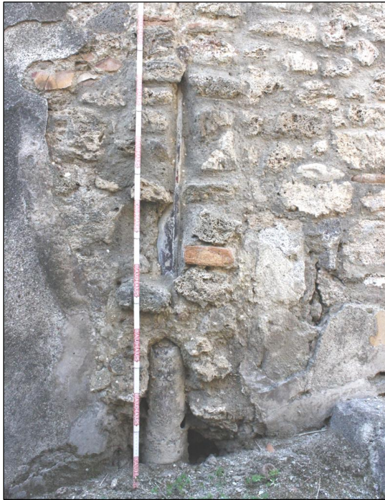
Figure 43A. A lead pipe is embedded in the W wall of Room 80 in Unit IX.3.15. Photo: author, 2011.
