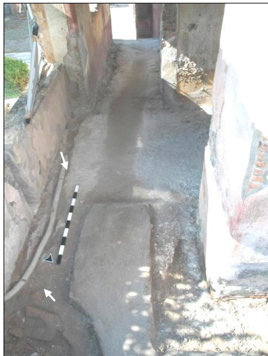
Figure 45B. The pipe runs in a groove made to the S edge of Rooms 20 and 21, and then turns to the garden (Room 18). Photo: T. Tuukkanen/ EPUH , 2004.
