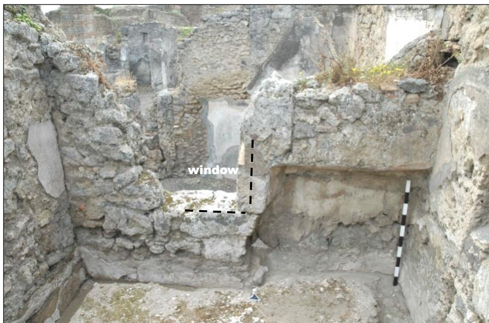
Figure 18B. The height of the window in the W wall of Room 135 (Unit IX.3.25) has probably been lowered thanks to the raising of floor levels. Photo: T. Tuukkanen/ EPUH , 2009.
