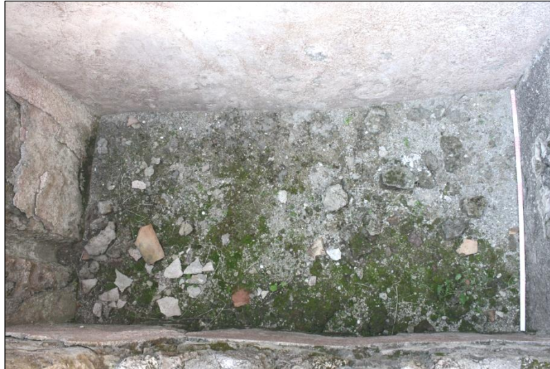
Figure 38A. A (former) water tank in Room 79, Unit IX.3.14. On the E wall (on the right), thick hydraulic plaster is replaced by non-hydraulic one. Photo: author, 2011.
