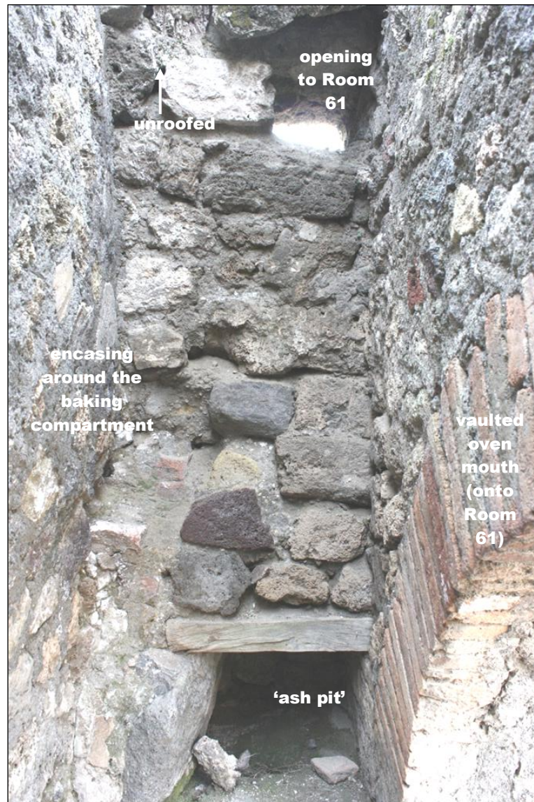
Figure 20. An unroofed space between the oven mouth and the baking compartment of the oven (Room 62) in Unit IX.3.10-12 contains an opening to Room 61. Photo: author, 2011.
