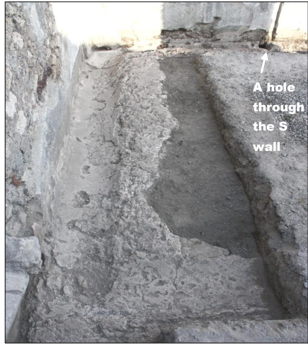
Figure 42A. A gutter along the E wall of Room 49-51 in Unit IX.3.1-2. Water in the gutter seems to have drained through a hole in the S wall to Room 54. Photo: author, 2009.
