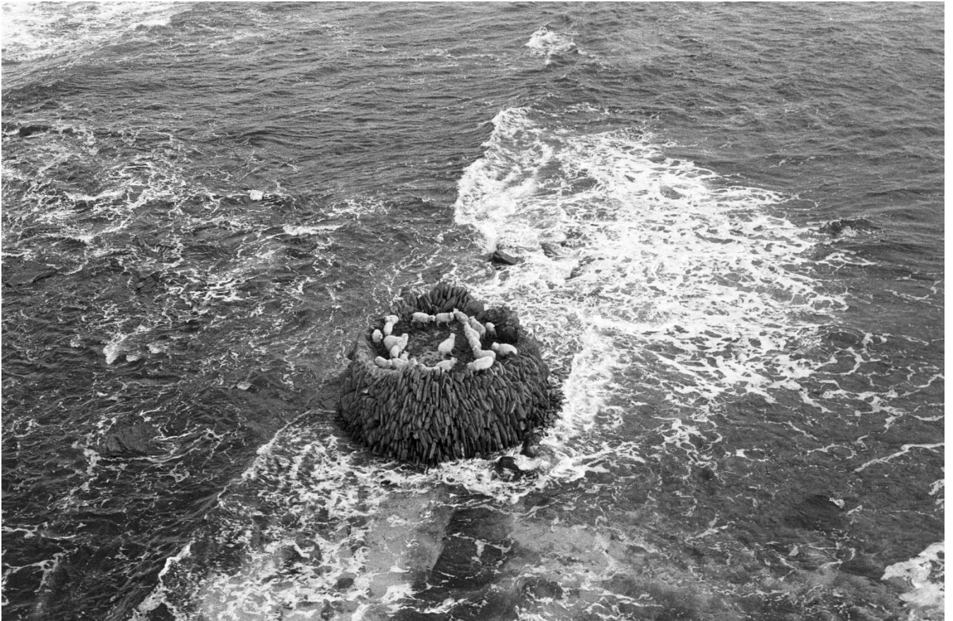
Fig. 2 Sheep fort in the North Atlantic Ocean, South of Rusk Holm, Orkney Islands. A human-built island (made of stone) for sheep to rescue themselves onto when cut off from land by the incoming tide. Picture taken by Gunnie Moberg, reproduced here with permission from Orkney Library & Archive.
