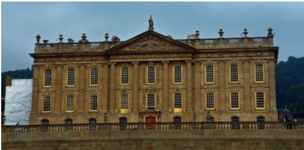
Fig. 4.9 Chatsworth House, west front (1700-1705) Image: Duncan Harris, Wikimedia Commons.
