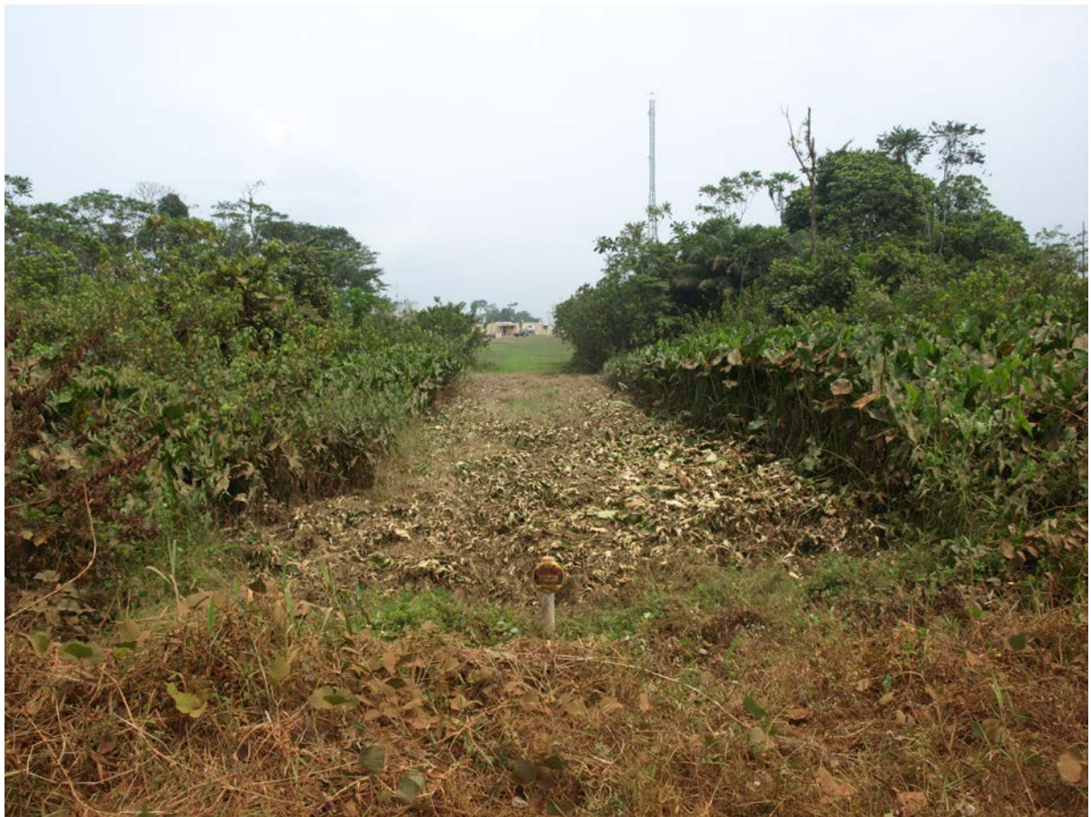
Figure 12. Recently cleared pipeline right-of-way, with pump reduction station visible in background. Near Mpango, outside Kribi, Cameroon.
