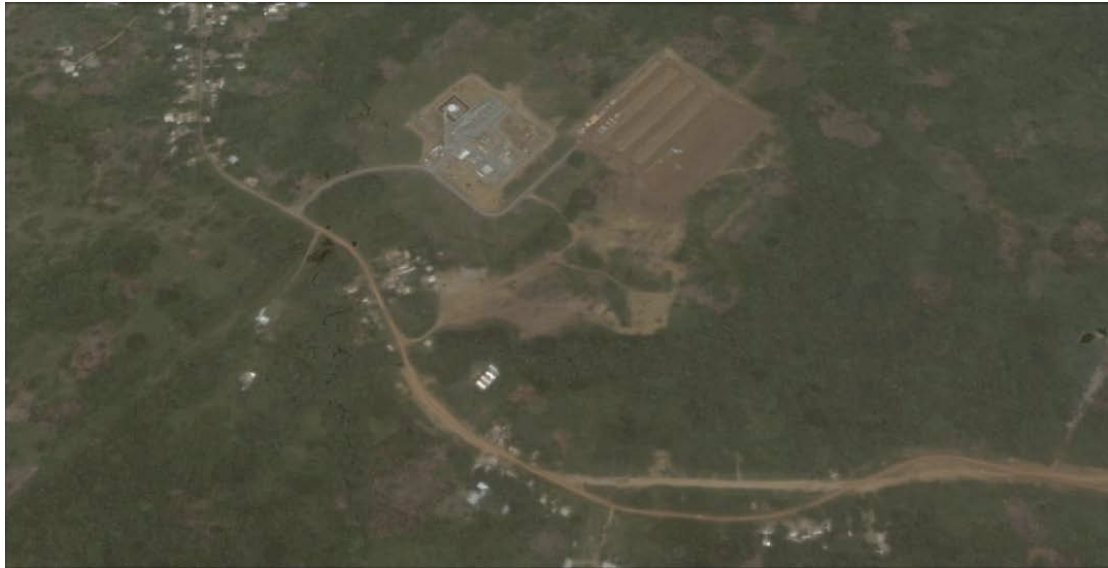
Figure 4. Pipeline Pump Reduction Station figures largely in the center of this image (note the two barren plots of earth). The village Mpango is to the southwest of the station. The southern edge of the community of Kribi is visible in the northwestern corner. Source: Google Earth.
