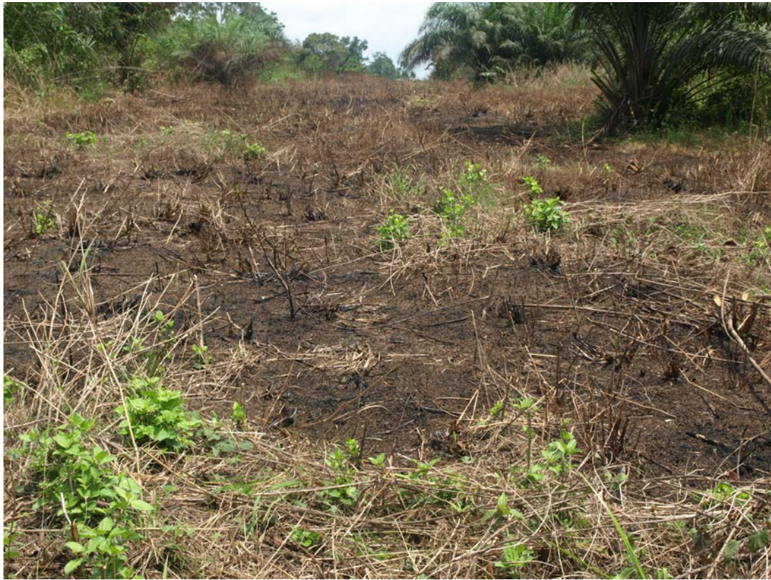
Figure 5. Recently cleared pipeline right-of-way, near Kribi, Cameroon.
