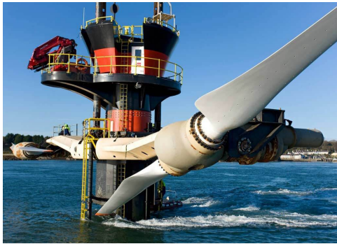
Figure 1.2: SeaGen turbines (Image reproduced with permission of Atlantis Resources.)
