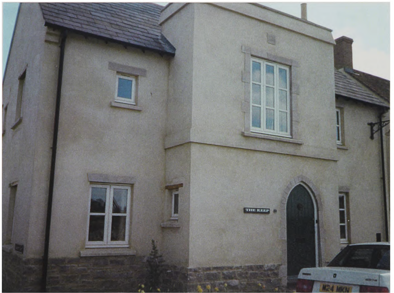
FIGURE 49: Density gradation, from compact terraces adjoining the central square (top); to larger detached houses on the quarter's periphery (below)
