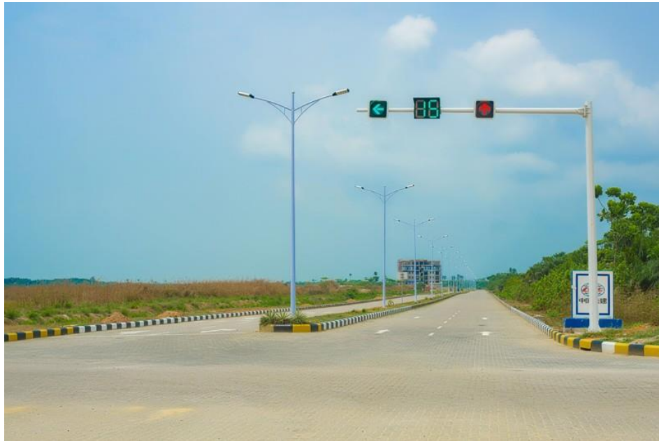
Figure 16: Road network within the LFTZ
