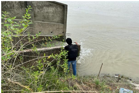
Residential wastewater discharge
