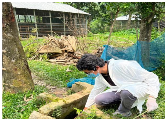
Drain near the poultry farm
