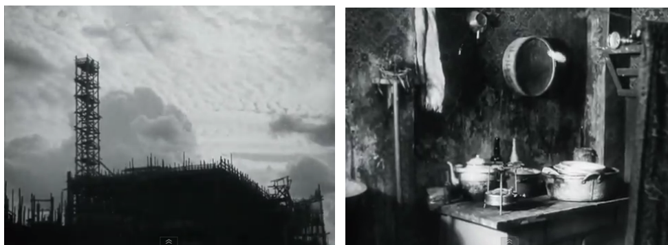
Figures 25 and 26. Tret'ia Meshchanskaia . The construction site and the kitchen.
