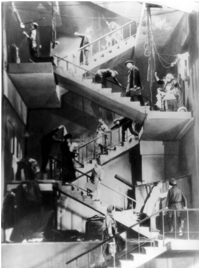
Figure 41. Dom na Trubnoi . The staircase.
