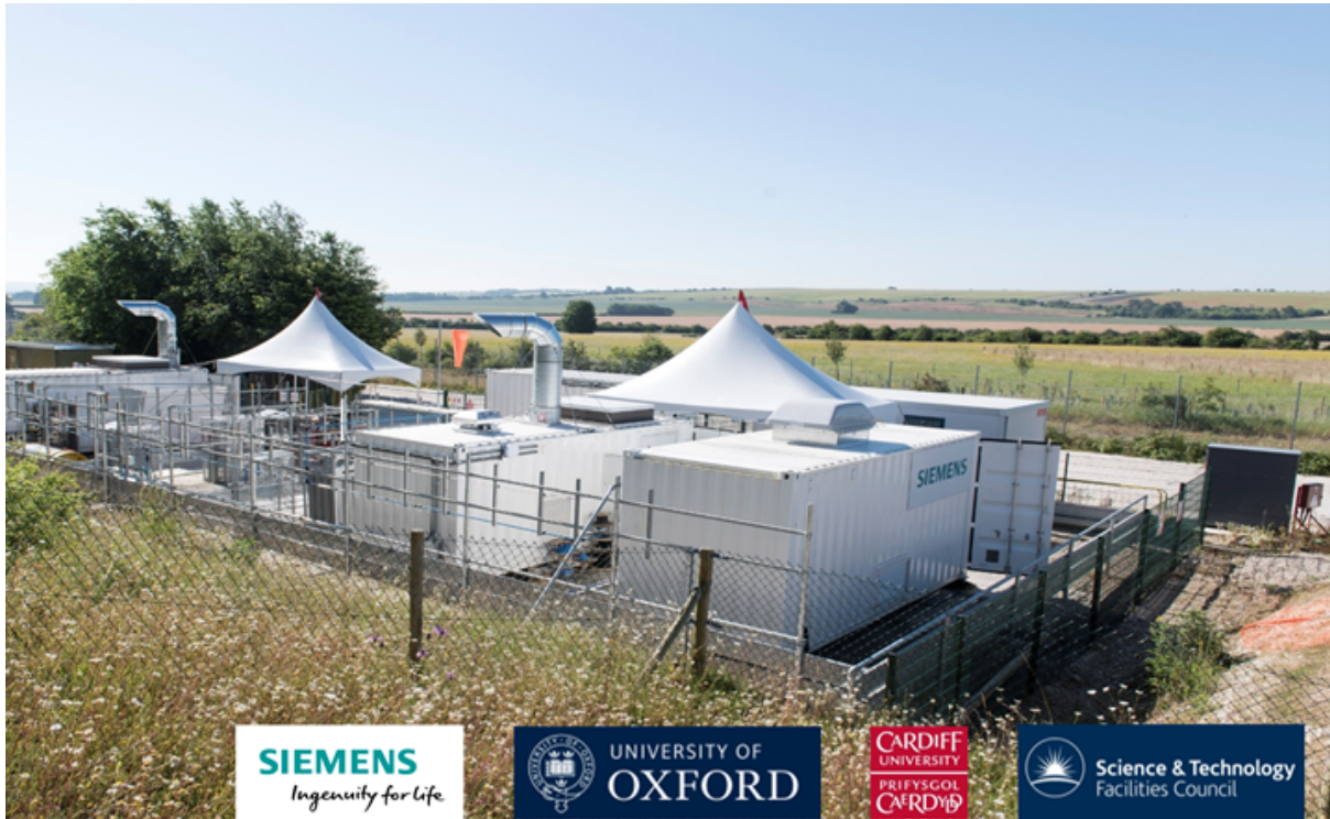
Figure 1.2: Power-to-ammonia-to-power demonstrator built at Rutherford Appleton Laboratory in Oxfordshire, UK as a collaboration between Siemens, University of Oxford, Cardiff University, and the Science and Technology Facilities Council (STFC). The system includes wind power, electrolysis, air separation via PSA, Haber-Bosch ammonia synthesis, ammonia storage, and ammonia / hydrogen combustion in a reciprocating engine.
