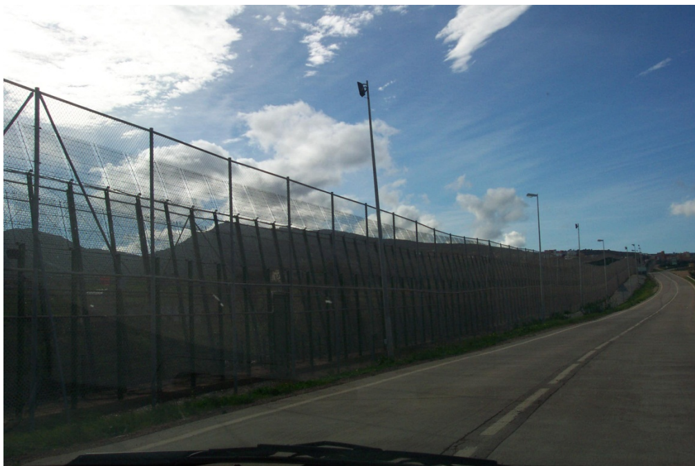
The new fence built in 2005 is 10 km long.
