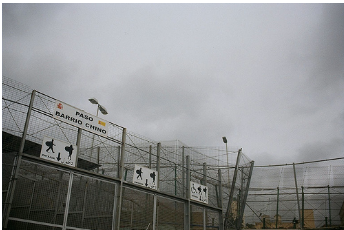
The signs on the fence indicate which doors are to be used by smugglers. Source: Prodein. 34
