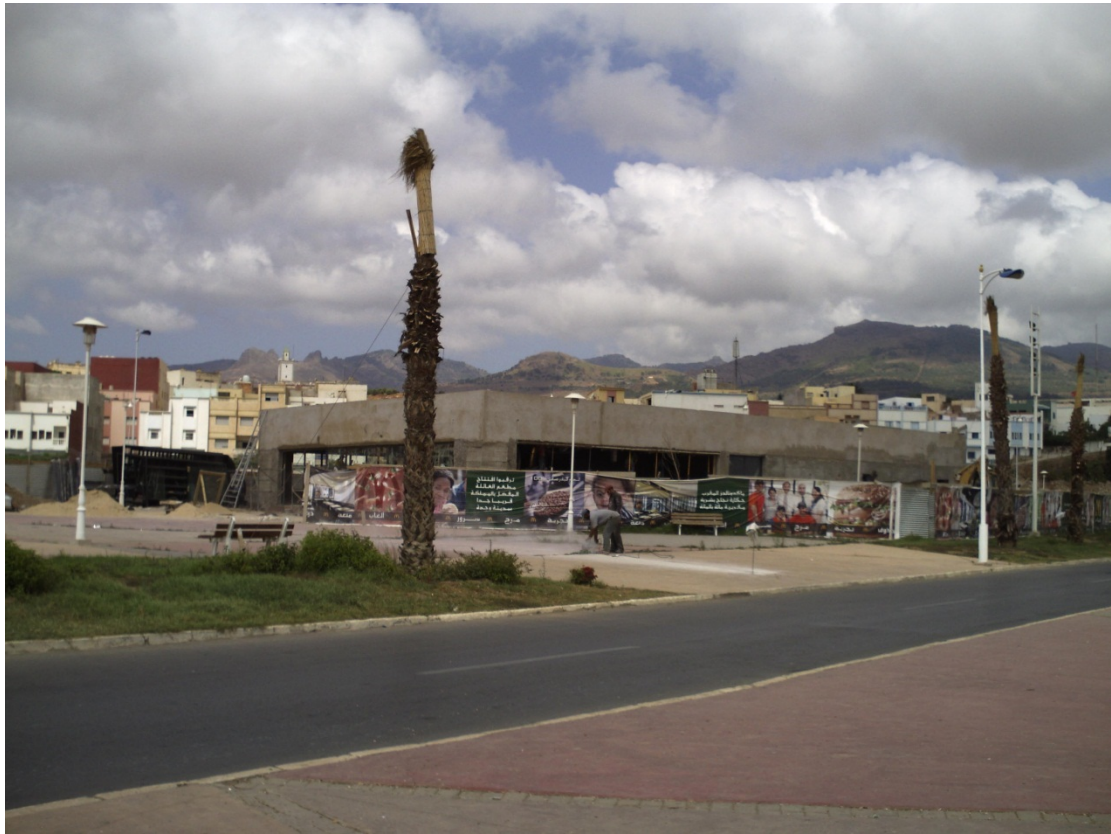
MacDonald's construction site in Nador
