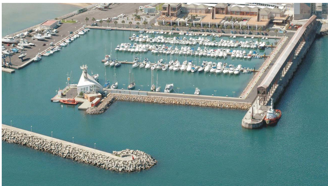
Extension of the port
