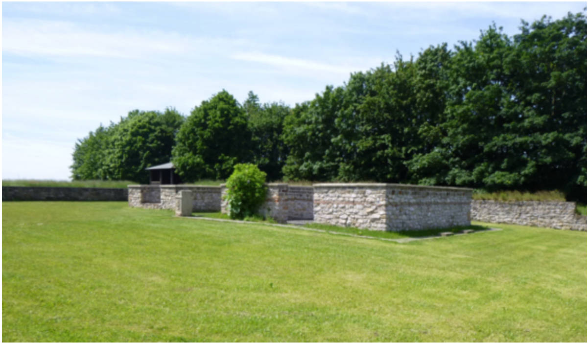
Figure 3.25: Modern reconstruction of the temple site at Nettersheim.
