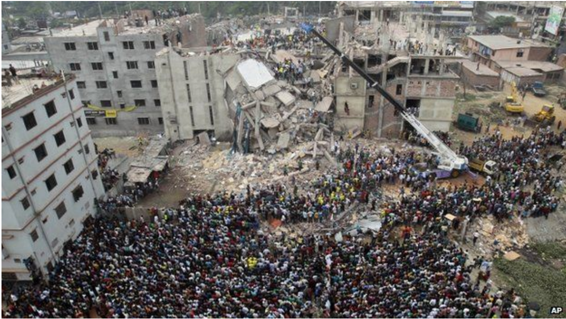
Figure 6: On 24 April 2013, an eight-story building known as Rana Plaza collapsed in Bangladesh, killing 1,134 individuals. It is considered the deadliest garment factory accident in history.
