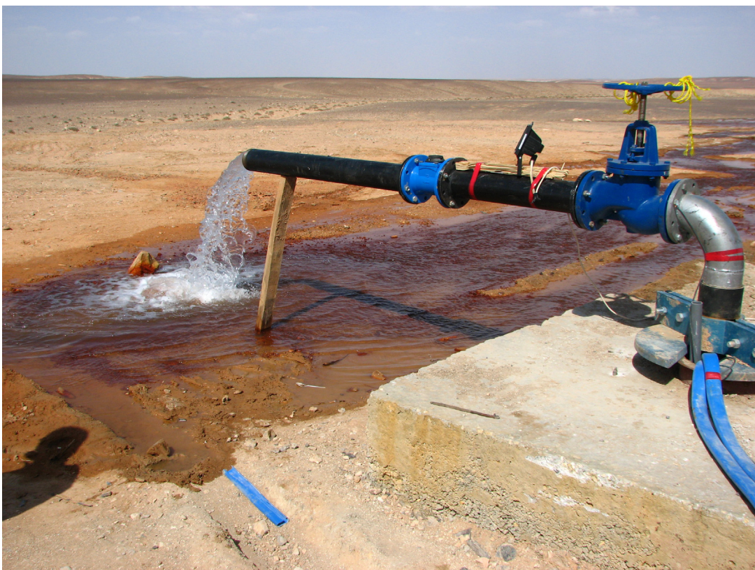
Figure 28 Test drilling of groundwater in Jordan.
