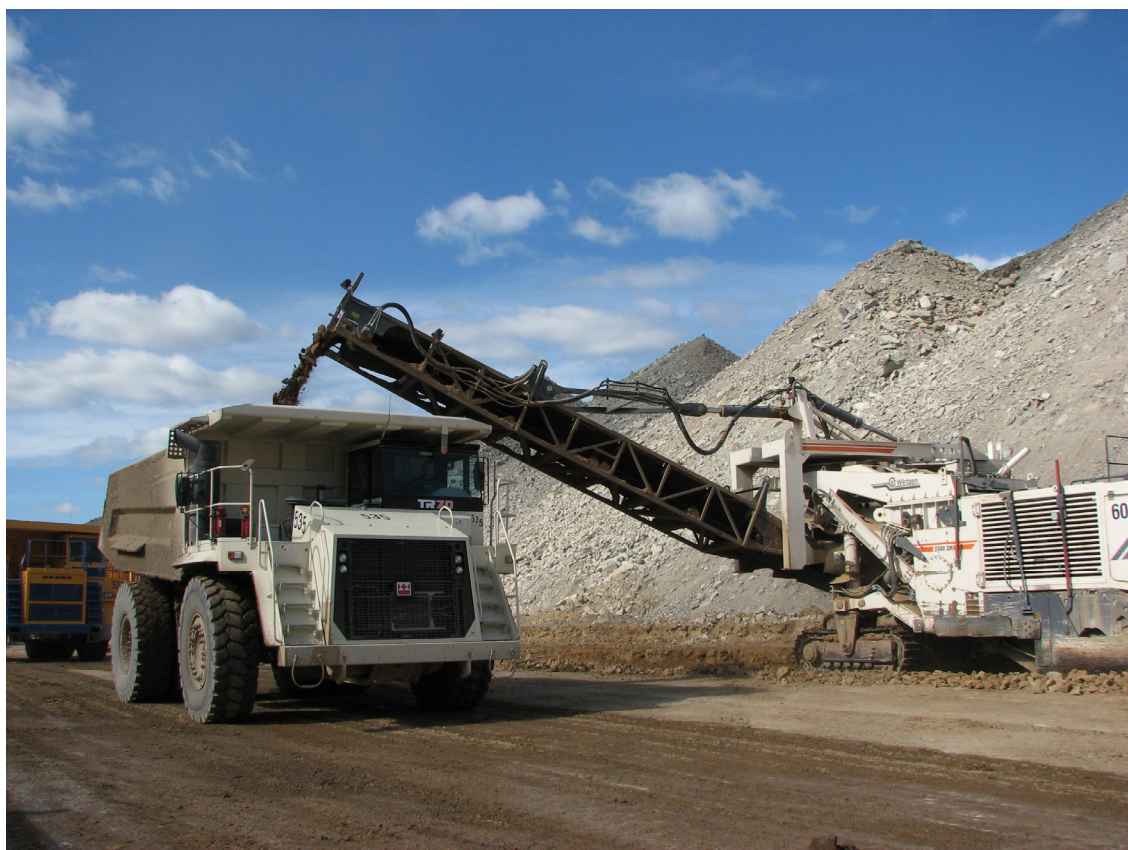
Figure 9 Selective mining with a terrain leveller in Narva quarry.
