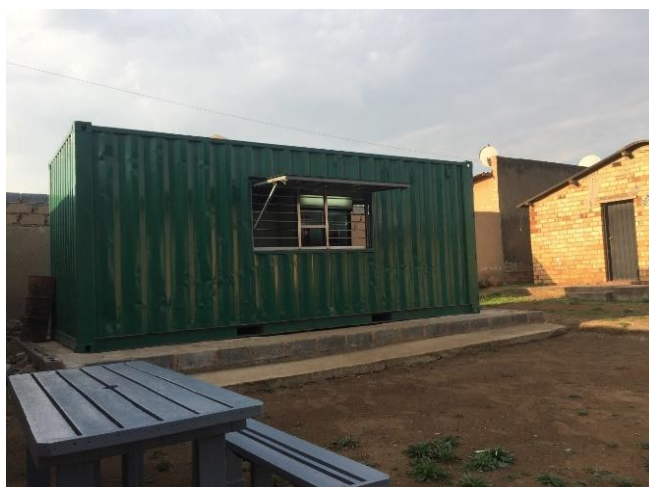
Figure 7: Container structure – food-preparation facility
