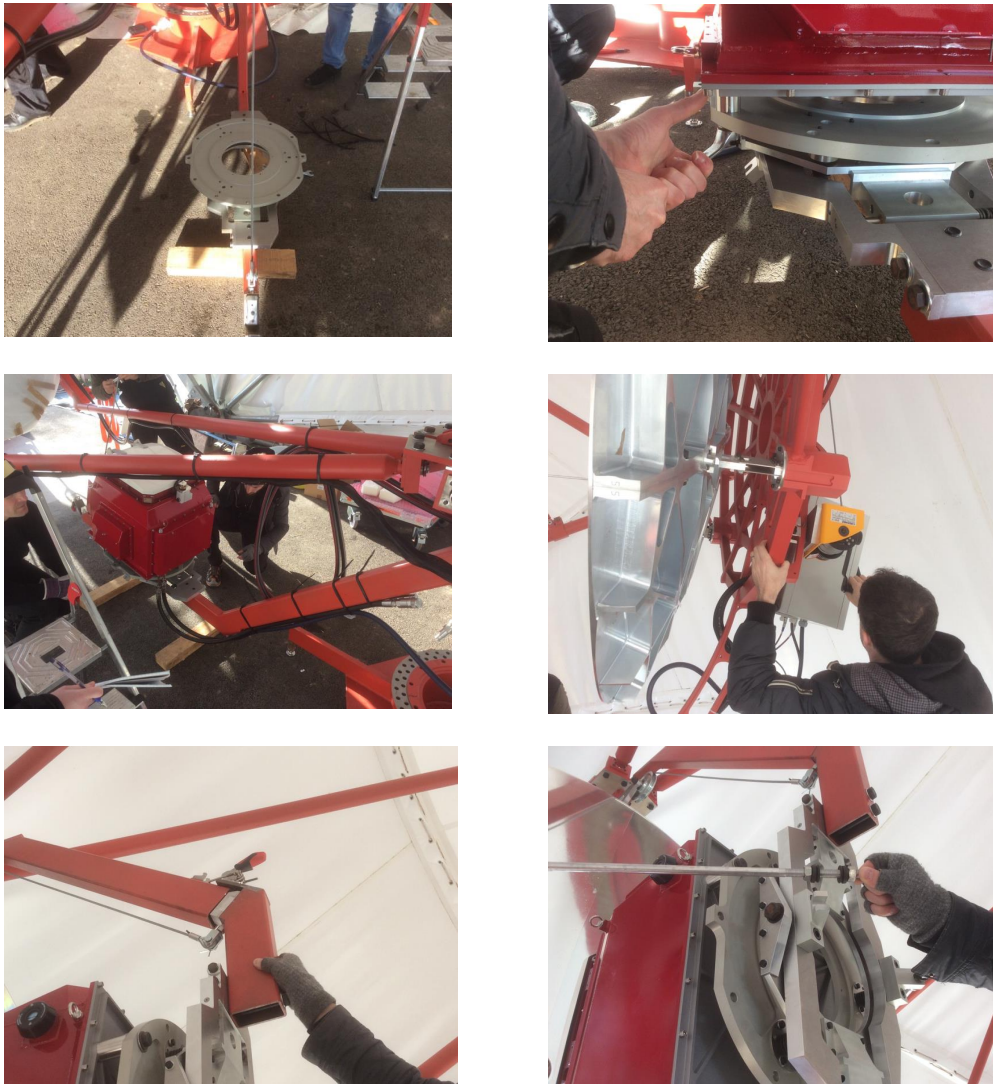
Fig. 5.5 Mounting procedure of the camera to the telescope structure. From left to right, top to bottom. (1) Lower the arm of the structure to host the camera to ground level. (2) Securing the camera with three bolts. (3,4) Raising the arm with the camera with the help of a winch on the rear of the secondary mirror. (5) Latching the arm with rest of the structure. (6). Securing the two horizontal support arms. These remove vibration of the camera and help stabilize the position of the focal plane with respect to the secondary mirror.
